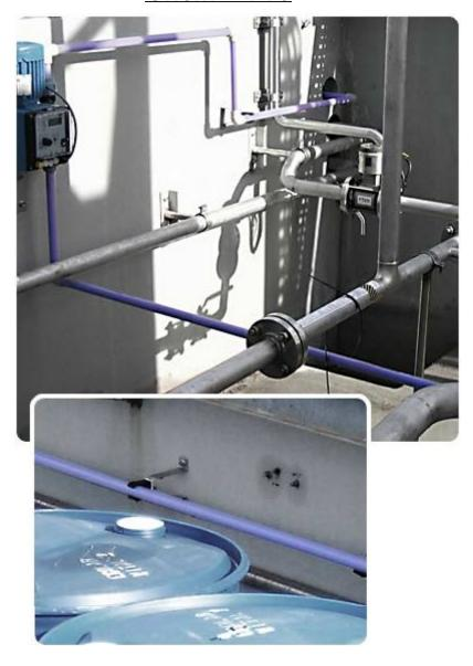
The Chem-Pro<sup>TM</sup> system is part of the family of safety-oriented colour-coded piping systems that conform with the requirements of standards relating to content identification of pipes, conduits and ducts, including AS1345 (1995).
